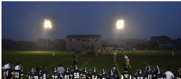
Existing Athletic Field Lighting
